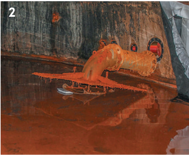
PICTURE 4 A new membrane is installed, flanges, suction fitting and other components are replaced. The tank is as good as new!
